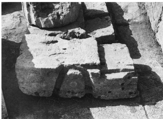
Fig. 5. Side of geison block G15 , with U-shaped channel for lifting and inserts in mutule
