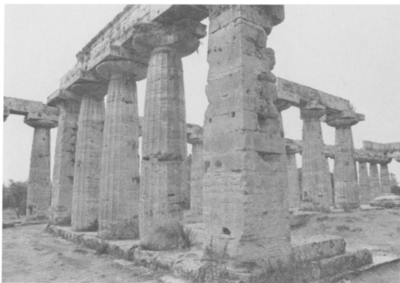
Fig. 4. Temple of Hera I, view of pronaos and interior colonnade.
