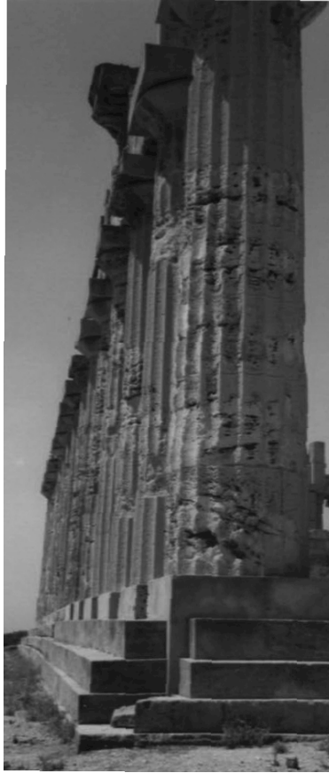
Fig. 11. The curvature of the stylobate of Temple of Apollo at Selinute, Sicily. Photo by the author
