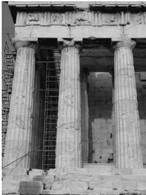
Fig. 10. Column entasis of the Parthenon in the context of adjacent columns. Photo by the author
