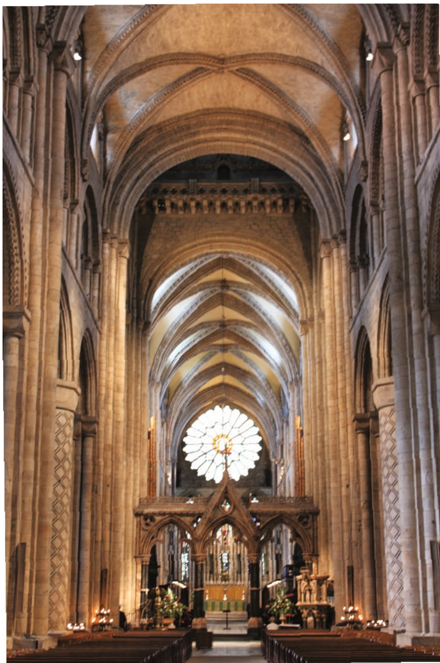
FIGURE 9.3 Durham Cathedral, vaulting of the nave AUTHOR'S PHOTO
