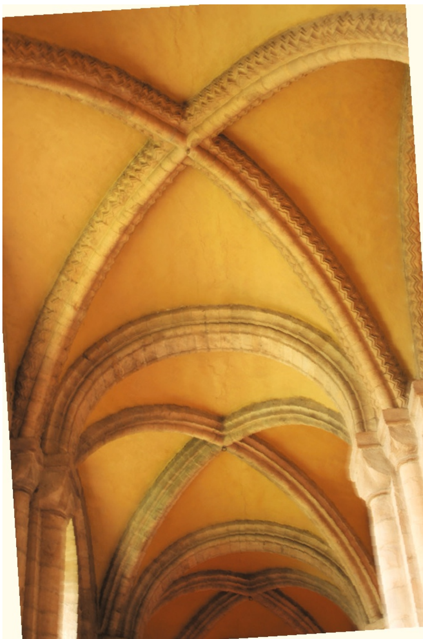
FIGURE 9.5 Durham Cathedral, arches and ribs in the choir aisles AUTHOR'S PHOTO
