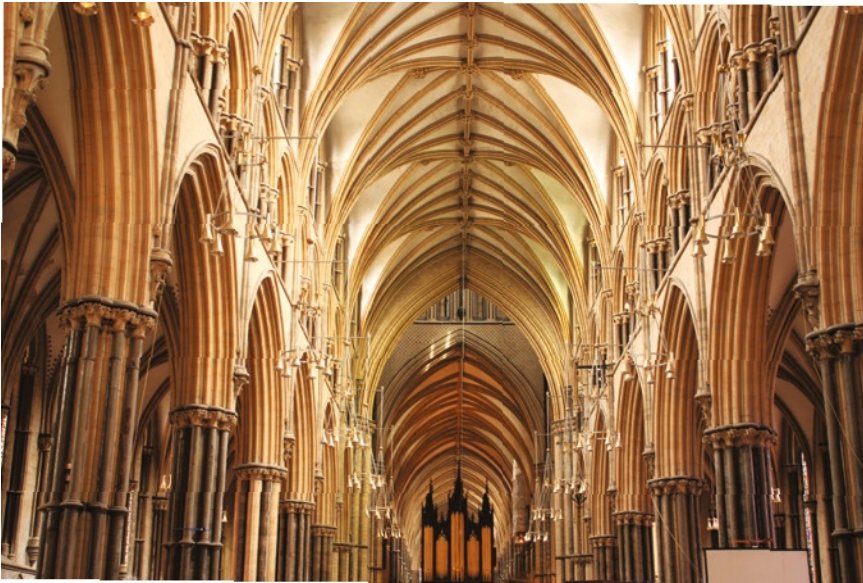
FIGURE 9.8 Lincoln Cathedral, vaulting of the nave AUTHOR'S PHOTO
