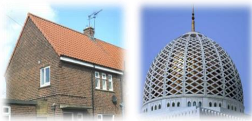
Fig. 6: Pitched Roof and Domed Roof Coverings.
